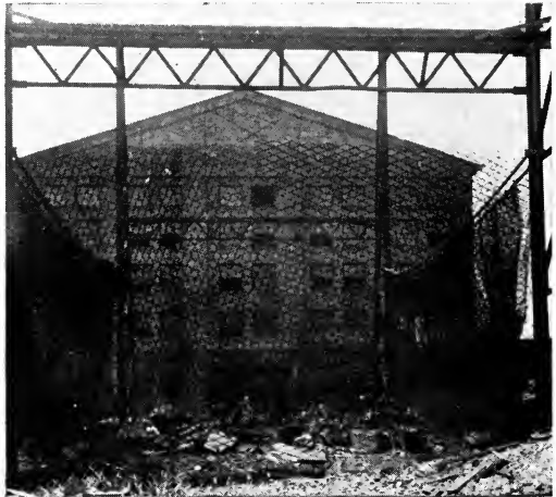
Candle-sticks that demand a good price are now made by the Reed and Prince Company from brass that was formerly thrown into the junk heap. The expense of broken windows and other damage caused by flying pieces was eliminated in one plant after the scrap-breaking yard had been penned in by three layers of expanded metal lath
